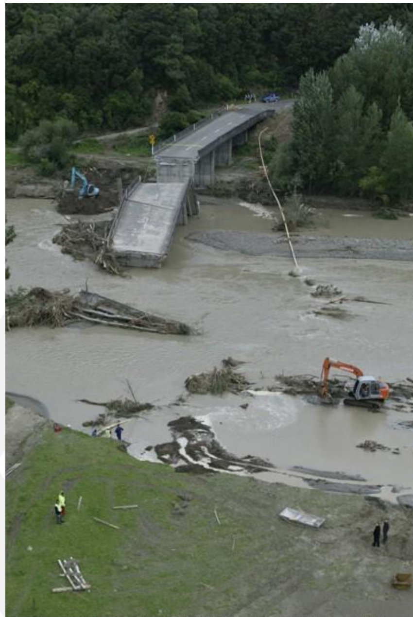
Saddle Rd bridge across Pohangina river with pipeline on right
